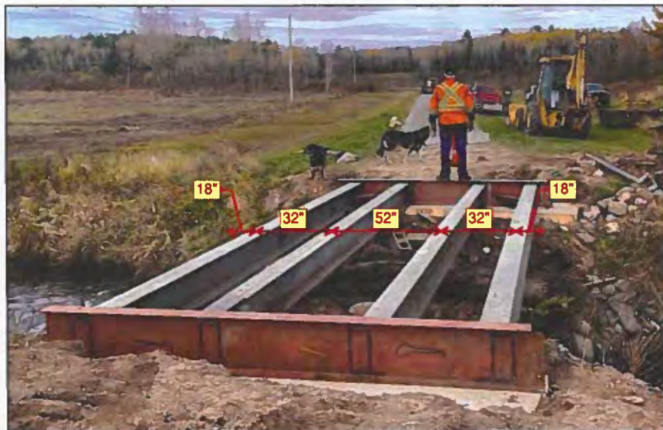
Photograph 1: Overview of Bridge (Under Construction)
