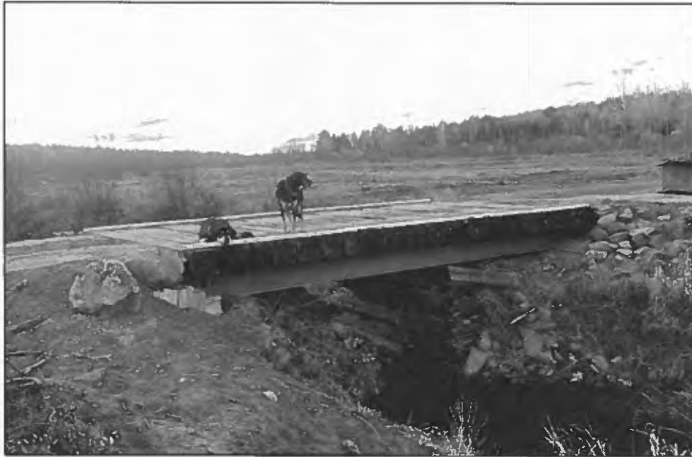
Photograph 2: Overview of Bridge
